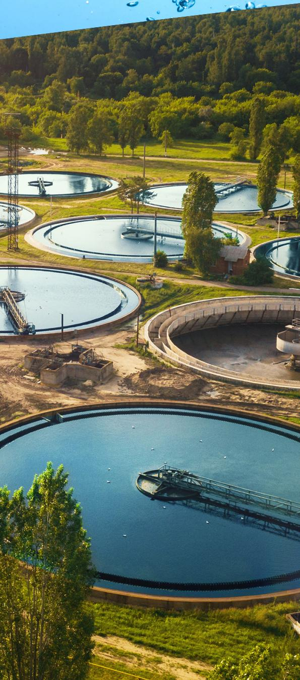
Biological wastewater treatment serves to break down excess nutrients such as nitrogen, carbon and phosphorus with the help of micro-organisms (activated sludge), thereby protecting water bodies from pollution. The nitrogen contained in the wastewater is eliminated in a multi-stage process.
